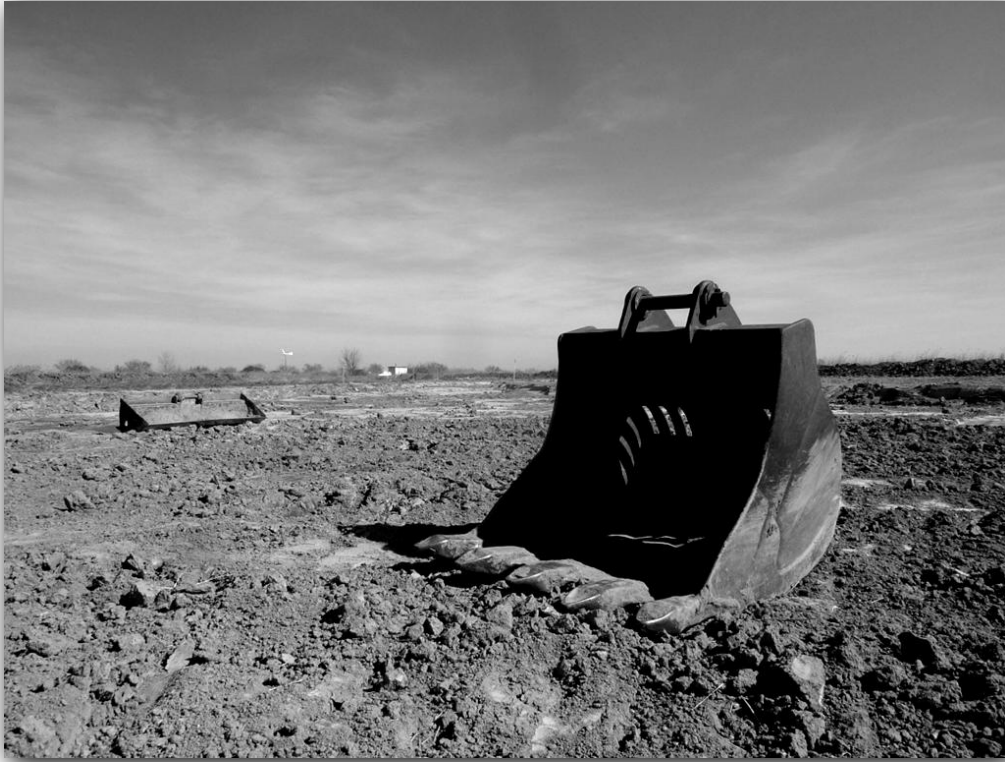
The Cassaïre site creation at large scale using a bulldozer to create topography.
