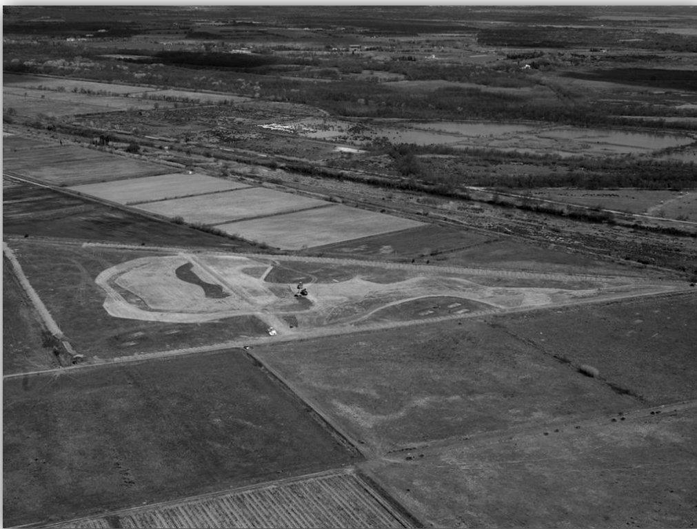
Aerial photography of the Cassaïre site during the creation (foreground the arable field, in background the wetland of the National Nature Reserve Les Marais du Vigueirat).
