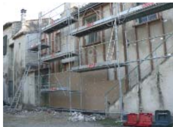
Installation of framework for insulation
