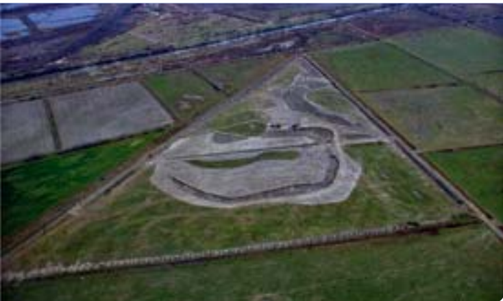
Engineering works on site
