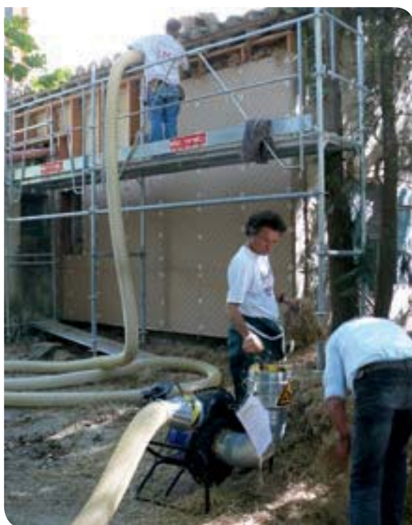
○ Filling-test of the formwork with rice straw
